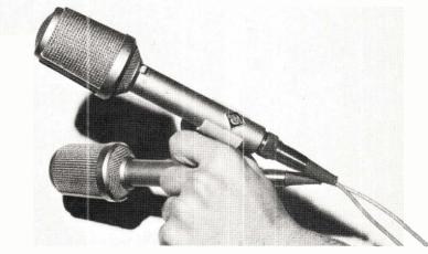
Crossed pair of Neumann KM 76 capacitor microphones — variable patterns set to cardioid — for location stereo recording.
